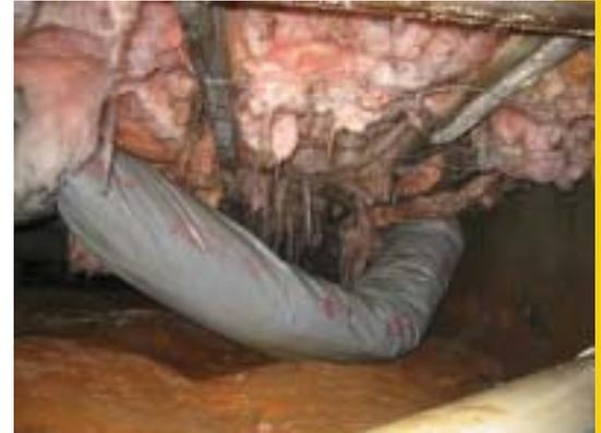
*Crawlspace with excessive moisture condensing on multiple cooler surfaces.*
